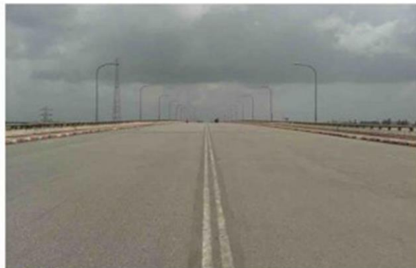
3 THANLYIN BRIDGE - 2 ( 20 mins )
