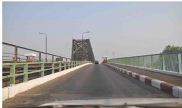
2 THANLYIN BRIDGE - 1 ( 30 mins )
